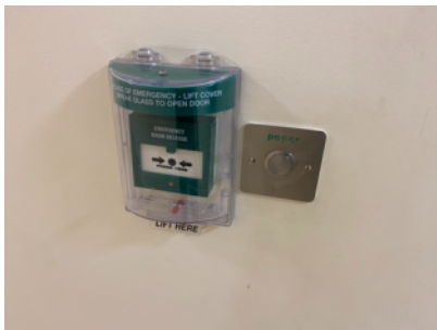
Electromagnetic door release & emergency door release at main entrance door
