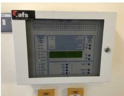
Fire detection panel
