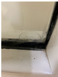
Acid etching visible on staircase door glazing.
