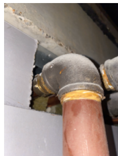
Pipe penetration without adequate fire stopping within riser cupboards.
