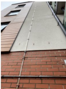
A lightning protection system is installed.
