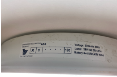
Non-maintained emergency lighting luminaire.
