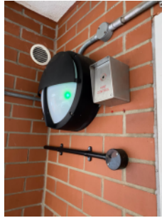
External non-maintained emergency lighting luminaire.
