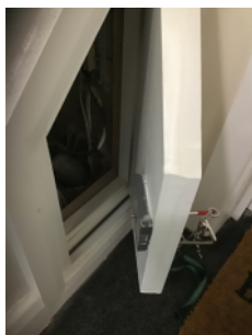
FD30S door to the electrical cupboard
