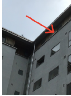
Timber cladding on sixth floor
