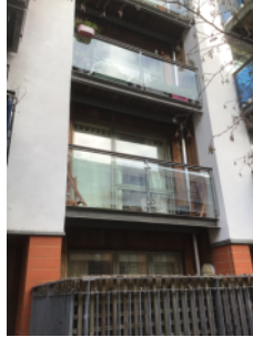
Timber cladding within inset (Juliet) balconies
