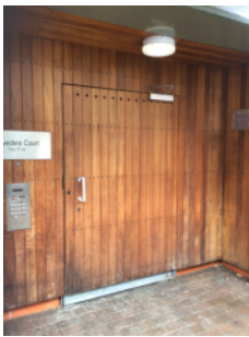
The externally accessed bin store was found locked and secured.
