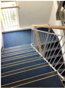
Escape route with contrasting stair nosings
