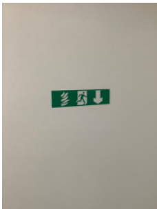
Escape route signage is provided
