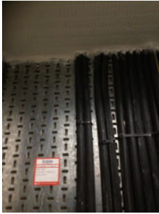
Fire stopping in risers and service cupboards
