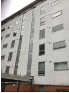
External walls end rear elevation
