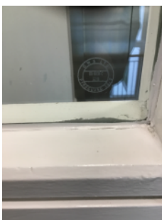
Acid etching on “Pyroguard” FR Glazed lobbies.
