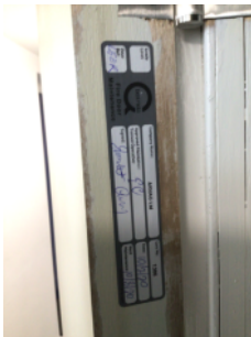
Evidence of riser door inspection in February 2020 by “ARVAG Ltd”
