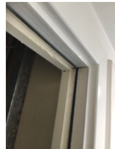
Intumescent strips and cold smoke seals fitted in riser cupboard doors.
