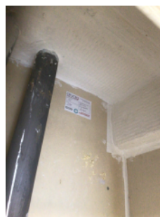
Fire stopping within riser cupboards
