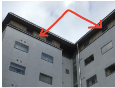
Showing timber cladding fitted on the sixth floor external walls.
