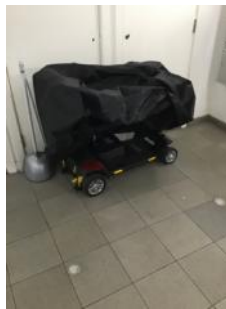
Motor scooter in ground floor escape route
