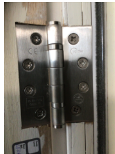
Standard of door hinge fitted in riser cupboard doors
