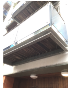
Private balconies – steel frame with timber deck glazed upstands.
