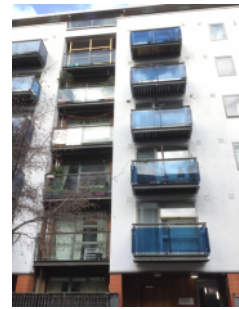
External walls – front elevation
