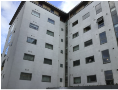
External walls - rear elevation
