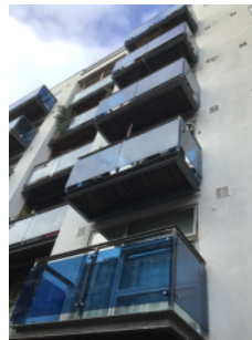
Configuration and construction of private balconies on the front elevation of the building
