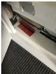
Fire stopping within electrical meter cupboards.
