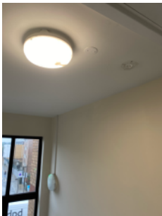
Maintained EL is provided in the staircase
