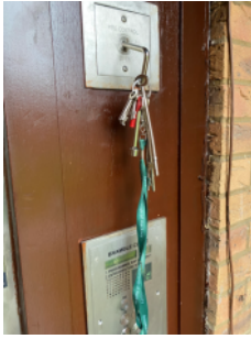
Entrance door override tested and found to operate correctly
