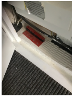
Fire stopping within electrical meter cupboards.
