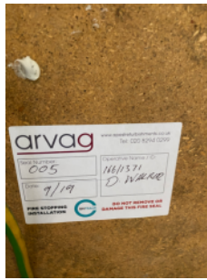
Example of fire stopping certification label in meter cupboards
