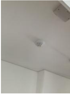
Heat detector in flat hallway
