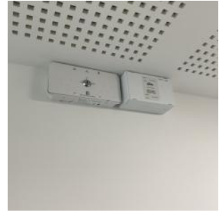
Radio link into each flat
