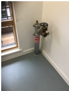
Dry riser outlet on staircase landings.
