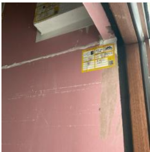
Evidence of fire stopping in riser cupboards
