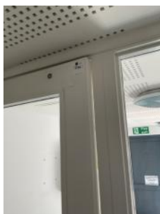
Ground floor lobby fire door does not close fully.
