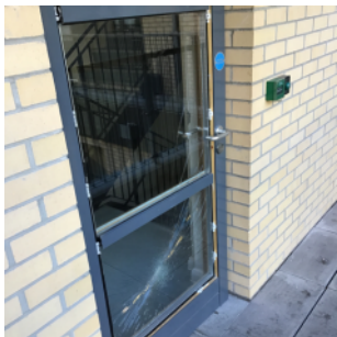
Version 5 - damaged fire exit door (V6 now completed)
