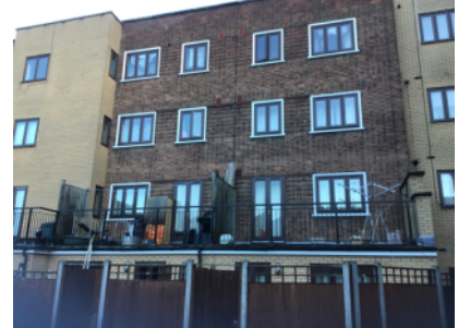
Rear elevation- brick/mortar walls, private balcony on 1st floor.
