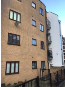
Brick/mortar external walls, with rendered section around the staircase External wall details
