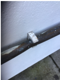
Gas pipe being damaged by the main entrance door
