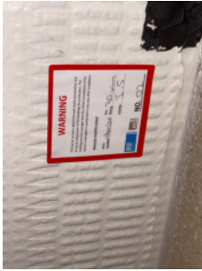
Fire stopping certificating label in riser cupboards.
