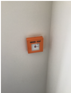
Smoke vent manual override switch.
