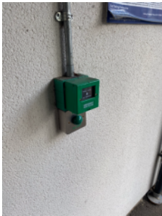
Electromagnetic gate release with emergency device.
