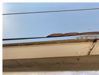
A damaged area exposes the core of the laminate EWS on front elevation.
