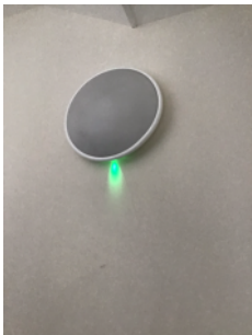
Emergency lighting in staircase
