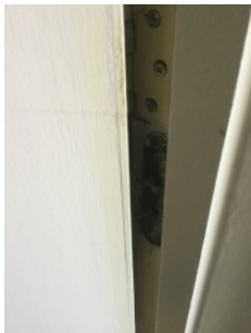
Concealed door jamb closer on entrance door to Flat A.
