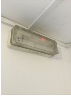
Non-maintained emergency light unit
