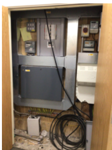
Main electrical intake and landlord's distribution board
