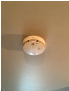
Interlinked hallway smoke alarm, flat 28
