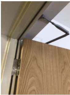
Self closer with intumescent strips and seals, staircase lobby
