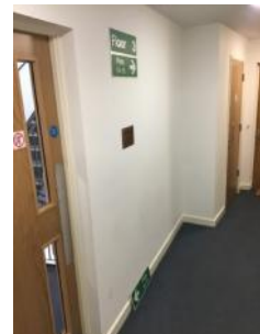
Wayfinding signage has fallen off the wall.
