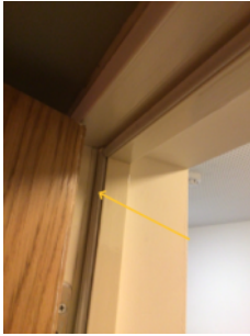
Flat 28- possibly surface mounted smoke seal
