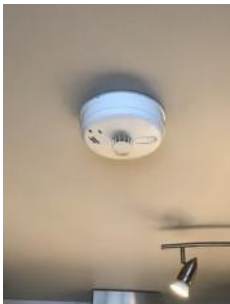
Interlinked kitchen heat alarm, flat 28
