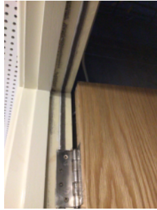
Intumescent strips and cold smoke seals installed on smoke shaft doors
