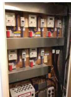
Electric meters in riser cupboard
