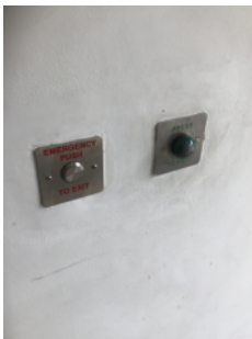
Door exit device with additional emergency exit device
