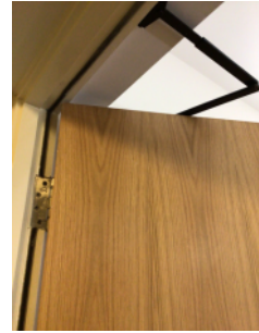
Self closer with intumescent strips and seals
