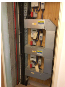
Electrical meters within riser cupboard
