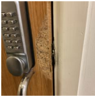
The left hand electrical cupboard fire door is damaged and requires repair.
