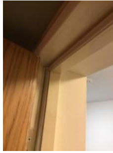
Example of believed surface mounted smoke seal
