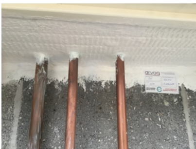
Evidence of recent fire stopping.
