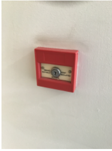
Smoke ventilation manual control located on the ground floor.
