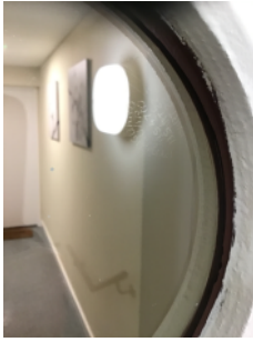
Staircase door glazing, showing “Pyroguard” acid etching
