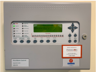
Panel for smoke detection for AOV actuation
