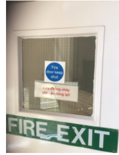
Georgian wired glazing installed in lobby doors
