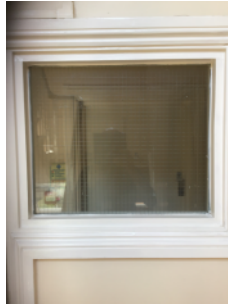
Georgian wired glazing installed in lobby partitions
