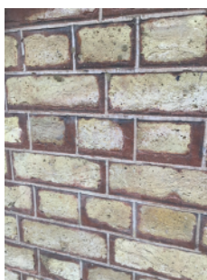
Original brick/mortar external walls
