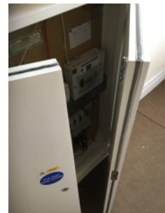
FD30S doors fitted to the electrical cupboard.
