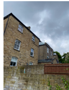
External walls - rear elevation
