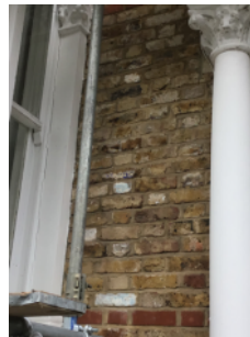
External walls are of the original brick/mortar construction.
