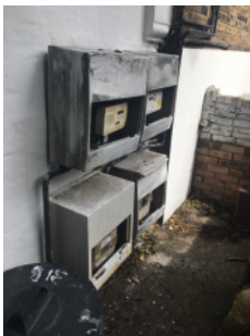
Gas meter cabinets- require repair
