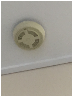
Part 6 smoke alarm in ground floor hallway.
