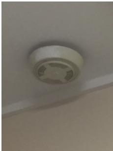
Part 6 smoke alarm in staircase.
