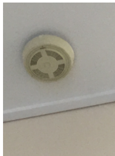
Part 6 smoke alarm on ground floor.
