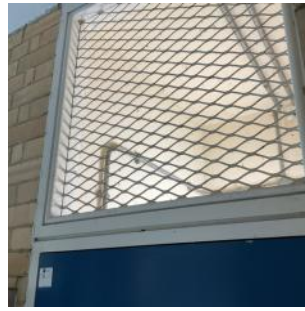
Vent above rubbish chute door
