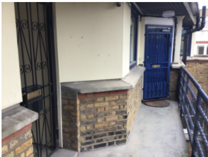
Security gates across flat entrance doors.
