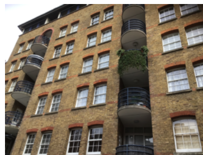
External walls – front elevation
