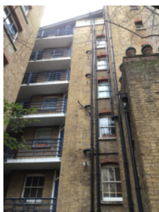
Brick/mortar external walls - rear elevation
