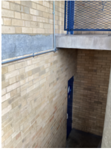
Brick / mortar walls with concrete floors in common areas
