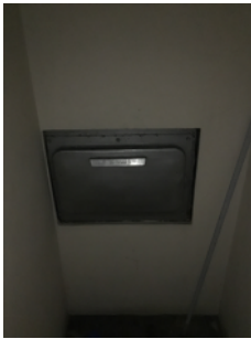
Example of rubbish chute hatch, in good state of repair.
