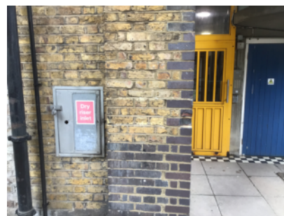
Dry riser inlet provided outside main entrance door.
