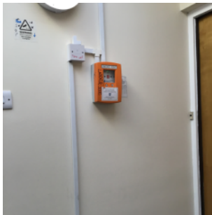
Smoke vent control panel
