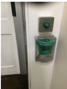
Door release and emergency door release.
