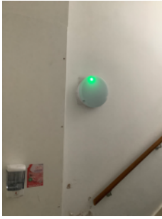
Maintained EL in the staircase
