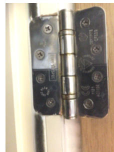
CE1121 Door hinges in riser doors.
