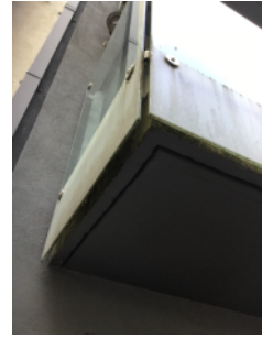
Common balconies- Concrete base with glazed up-stands
