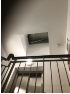
AOV Provided in the staircase
