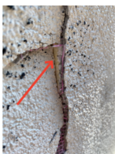
Insulated material beneath external rendered surface.
