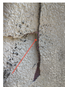
Showing insulated material beneath rendered surface.
