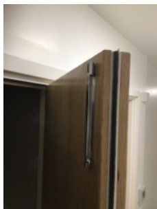
Intumescent strips and cold smoke seals installed in riser doors.
