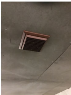
Breaches of the undercroft carpark ceiling
