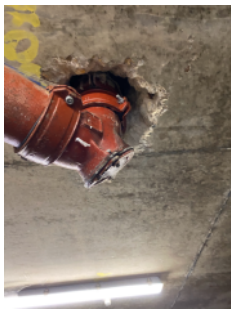
Pipe penetration through a concrete slab within the bin store.
