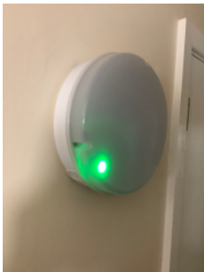
Maintained EL within corridors, and the staircase
