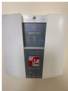
Smoke vent control – showing fault and alarm.
