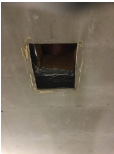
Breaches of the undercroft carpark ceiling
