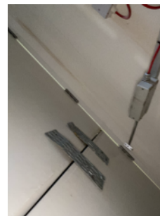
Opening mechanism at the rear of the smoke shaft door has become detached.
