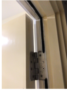
Strips and seals fitted to riser cupboard doors
