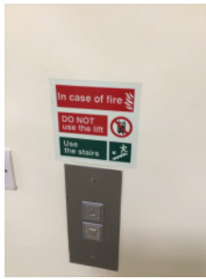
Suitable signage for lift
