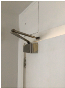
Overhead self closing device - flat entrance door
