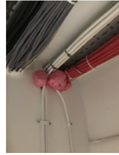
Pink intumescent expanding foam should not be used for large penetrations
