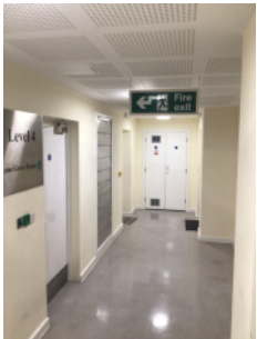
Escape route signage provided
