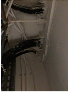
Evidence of fire stopping - riser cupboard on 6th floor
