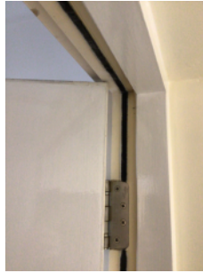
Strips and seal fitted to flat entrance door
