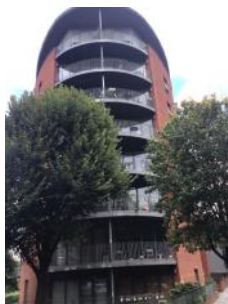
Combustibles noted on private balconies
