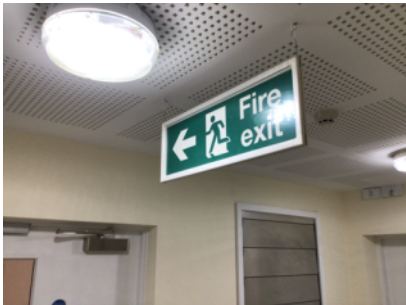
Escape route signage provided
