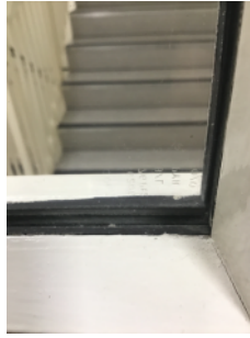
Acid etching on glazing.
