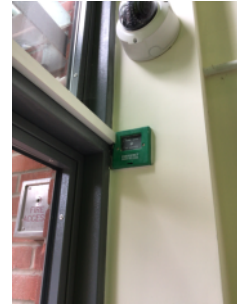
Green break glass emergency exit device
