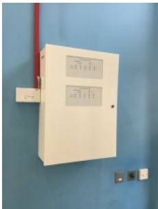
Original Part 1 system for AOVs
