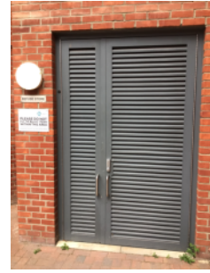
Secure waste bins store
