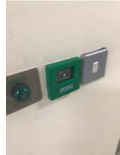
Green break glass unit to staircase / lobby door
