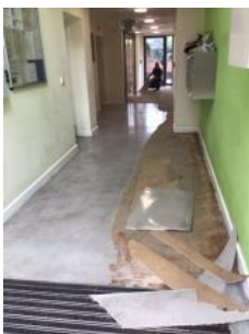
Contractor on site, replacing floor covering in entrance lobby
