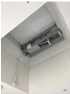
AOV at head of staircase
