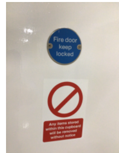
Suitable keep locked signage displayed on riser doors
