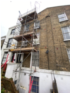
Scaffold erected on front face of building
