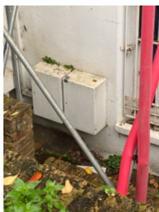
Gas meters located externally
