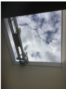
Smoke vent in roof open
