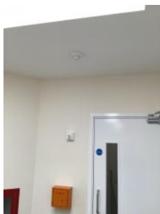
Smoke detector within staircase
