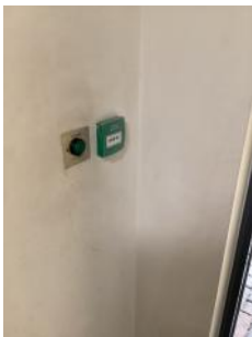
Push to exit button with emergency override at front entrance
