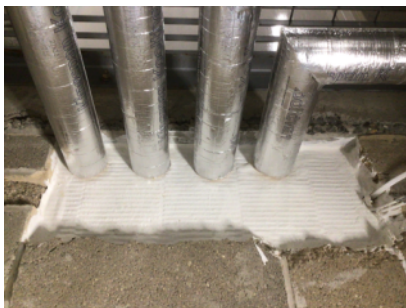
Standard of fire stopping installed in riser cupboards
