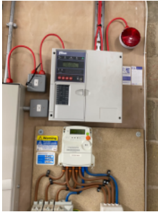
Fire alarm control panel in plant room
