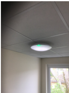
Emergency lighting provided in corridors and staircase.
