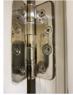
Fire door hinges to BS EN1935 standard
