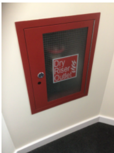
Dry riser outlets in staircase
