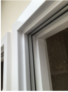
Intumescent strips and cold smoke seals installed in riser cupboard doors.
