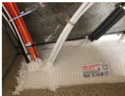
Standard of fire stopping installed in riser cupboards
