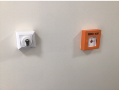
Manual smoke vent controls
