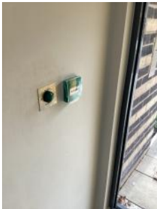
Press to exit with emergency override at front entrance
