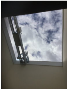
Smoke vent in roof open
