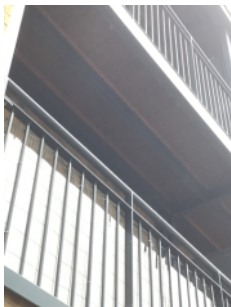
Private balconies-steel framed with timber deck
