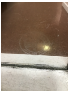
“Pyroguard” FR Glazing in corridor doors.
