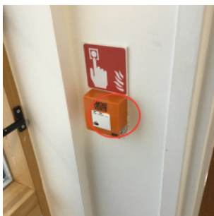
Fault light on smoke vent actuator
