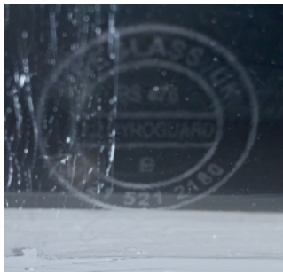
“Pyroguard” FR Glazing in corridor doors.
