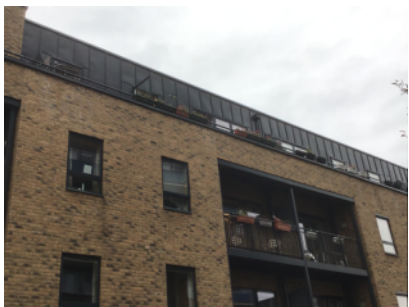
Metallic cladded external wall system on fourth (uppermost) floor.
