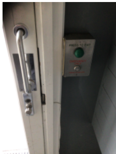
Electromagnetic door release mechanism with emergency override.
