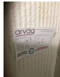
Fire stopping certifying label in riser cupboards.
