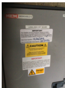
Evidence of testing of landlords distribution board.
