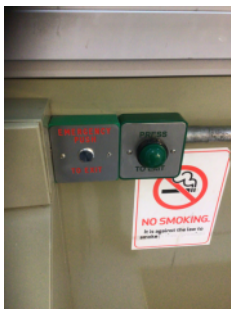
Electromagnetic door release and emergency door release, main entrance door
