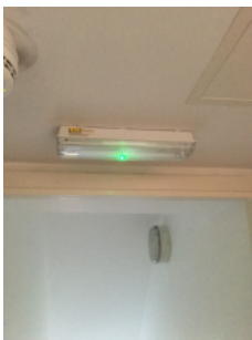
Non-maintained emergency lighting in staircase.
