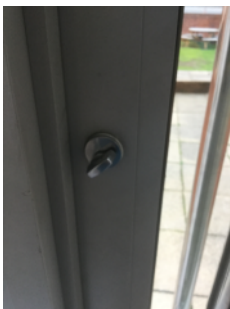
Thumb turn device on rear exit door.
