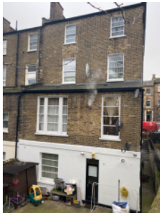
Rear elevation - original brick/mortar walls, with render to lower ground.
