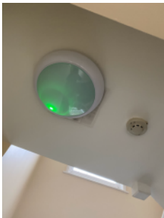
Maintained emergency lighting is provided in the staircase.
