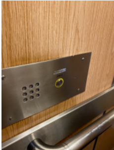
Telecare call-points are provided in the lift.
