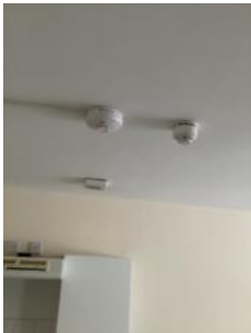
Heat alarm and detector flat 4 kitchen.
