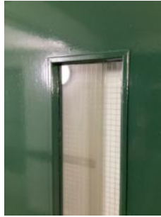
Georgian wired glazing in cross corridor door
