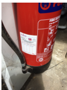
Dry powder extinguisher in boiler requires testing
