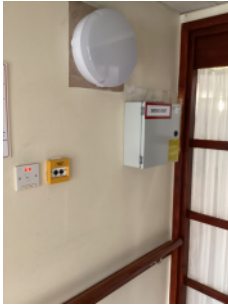
Smoke vent control and manual control
