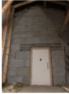
Compartmentation in roof space
