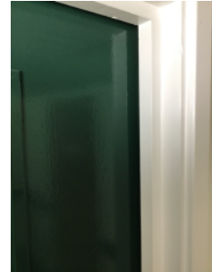
Corridor door not closing fully
