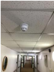
BS5839-1 detector and sounder in corridor
