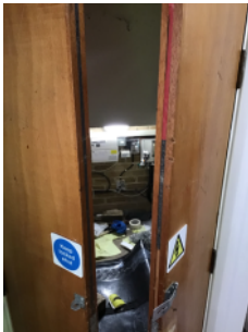
Combustibles in electrical cupboard
