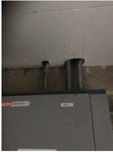
Cable penetrations within the electrical meter cupboard.
