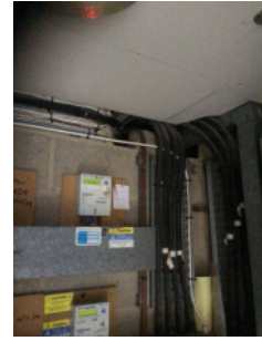
Cable penetrations within the electrical meter cupboard.
