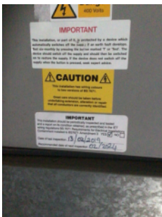
Evidence of inspection of electrical installations.
