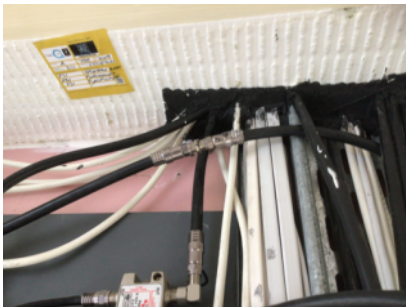
Fire stopping within riser cupboards.
