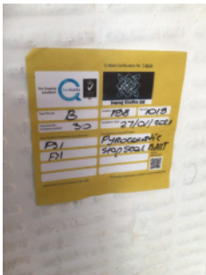
Fire stopping certificating label within riser cupboards.
