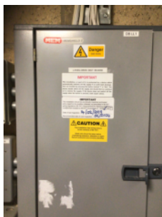
Evidence of testing of landlords distribution board
