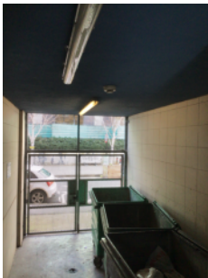
Bin store appears imperforate to the flats above (within scope of this FRA)
