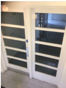
Georgian wired glazing on the staircase.
