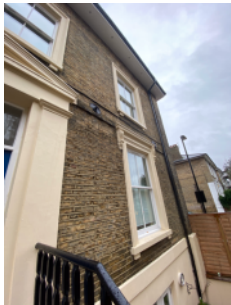
Brick/mortar external walls - front elevation
