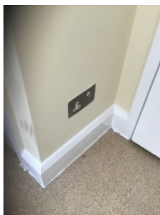
Electrical socket provided in common staircase
