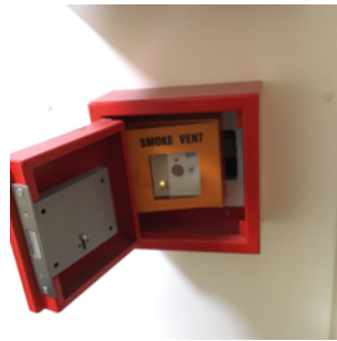
Smoke vent control showing a fault light
