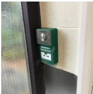
Exit release mechanism
