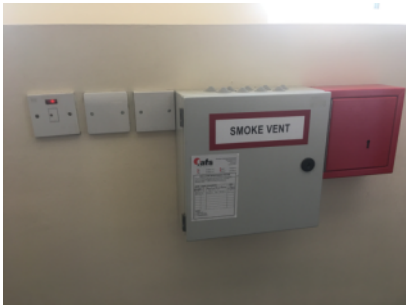
Smoke vent control panel.
