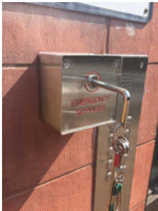
Entrance door override was tested and found to function correctly.
