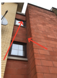
Indicating where it appears this section is a vertical hung tile system
