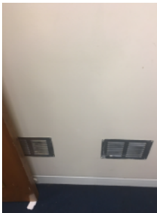
Confirm grill-vents are intumescent protected
