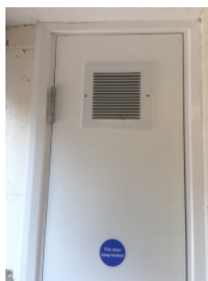
Vents in gas meter cupboard doors.
