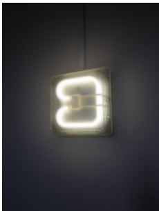
Maintained (local) emergency lighting provided in staircase
