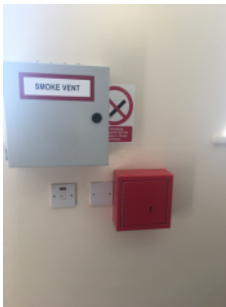
Smoke vent control panel.
