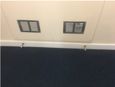
Confirm grill-vents are intumescent protected
