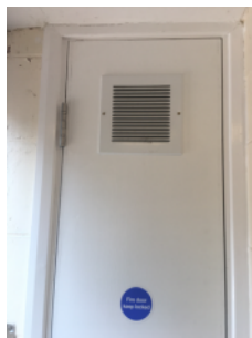
Vents in gas meter cupboard doors.
