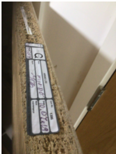
Fire door Certification on riser cupboard doors
