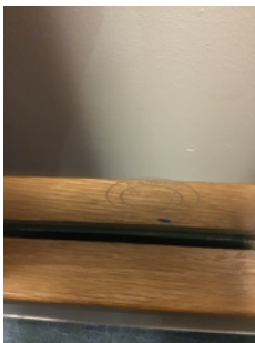
Acid etching on door glazing
