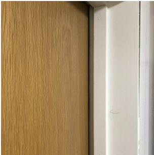
Ground floor corridor door not closing fully
