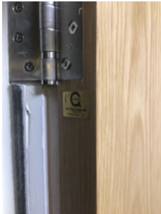
Fire door certificating on riser cupboard doors
