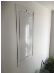
Smoke shaft door in the corridor
