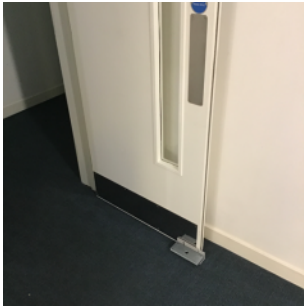
First floor staircase door wedged open
