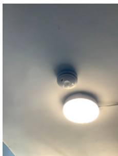
Part 6 fire alarm in common areas.
