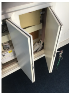
FD30S Doors fitted to the electrical cupboard
