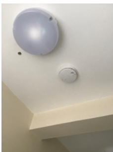
BS5839-6 fire alarm in the entrance hallway.
