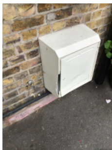
Broken gas meter cabinet.
