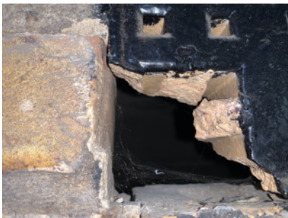
Broken grill above intake cupboard door.
