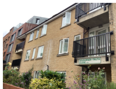
Brick/mortar external walls, with rendered section - rear elevation
