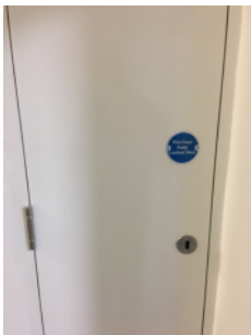
Fire Door Keep Locked signage on comms riser cupboard doors.
