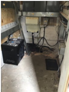
Combustible free electrical cupboard
