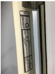
BMTrada door certification label on 6th floor staircase door
