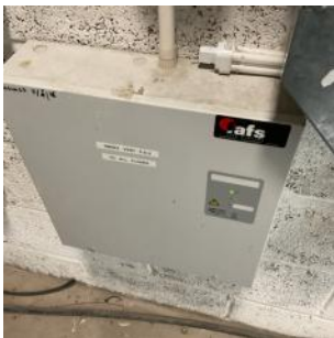
Smoke vent power supply unit healthy
