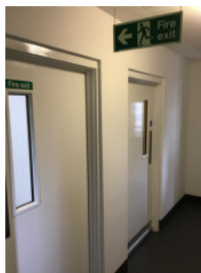
FD60S doors within lobby leading to the staircase and fire-fighting lift
