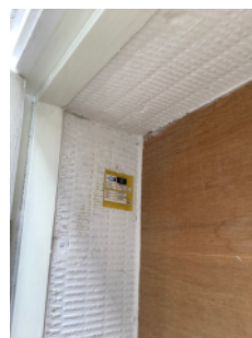
Fire stopping installed in riser cupboards
