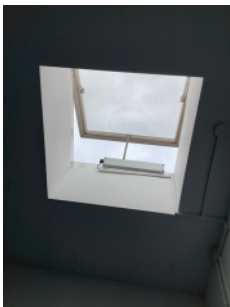
Staircase vent tested
