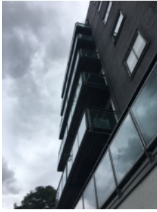
Private balconies - steel framed with glazed up-stands and timber decks
