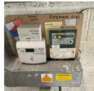
Separate power supply for firefighters lift
