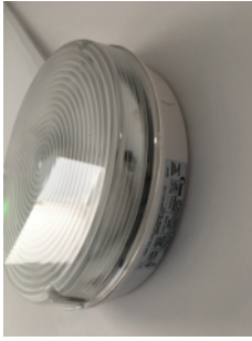
Emergency lighting unit in staircase
