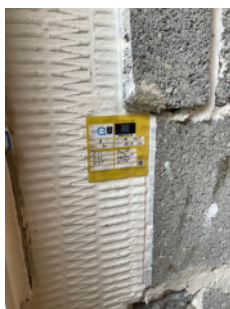
Fire stopping in riser cupboards installed December 2020
