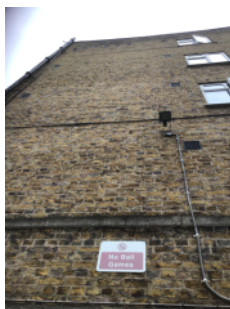
Original brick/mortar external walls
