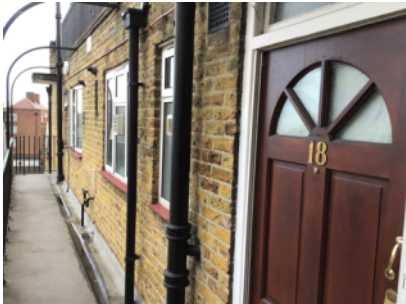
Fanlights and window glazing located above 1.1m
