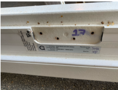
BMTrada QMARK certification label on NEW door frames being installed
