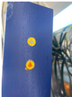
BWF Fire door identification plugs on the new door sets being installed
