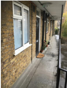
All glazing on common balconies above 1.1m
